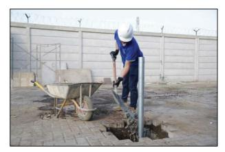
Step 7: Set the pipe vertical into the hole and start pouring the concrete.
